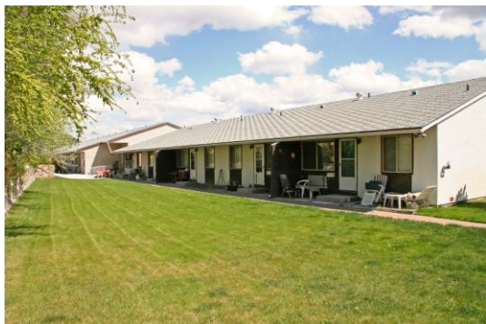
Thompson View Manor 15-Suite Independent Living Facility
