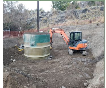
Lift Station #1 Chamber installed
