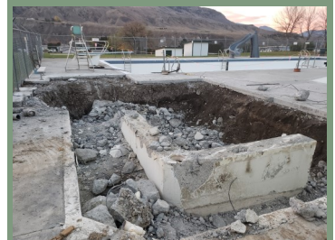
Hot Tub demolition
