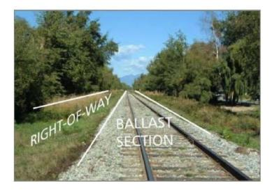
CN will use chemical control techniques on the ballast section and specific locations of the right of way throughout the network for safety reasons. Furthermore, when chemicals are applied via spray train or truck, additives called surfactants are included to make the chemical work better.
