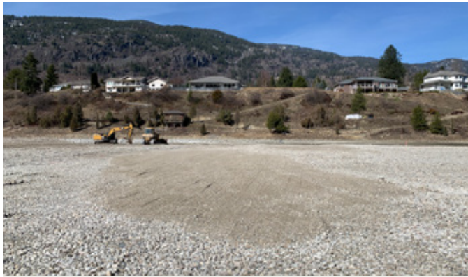
Recontouring in progress.
