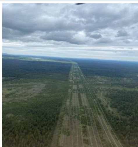
Figure 5. Fuel break linked to transmission line right-of-way
