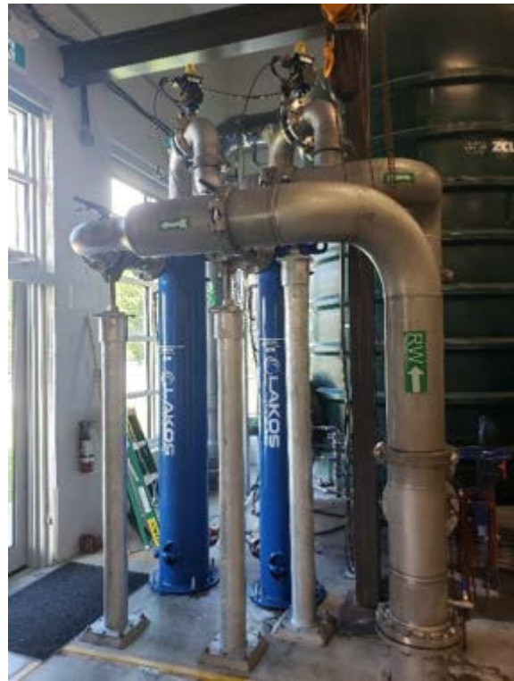
Below: Water Treatment Plant. Right: Sand separators
