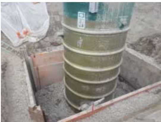
Lift Station installation (below)
