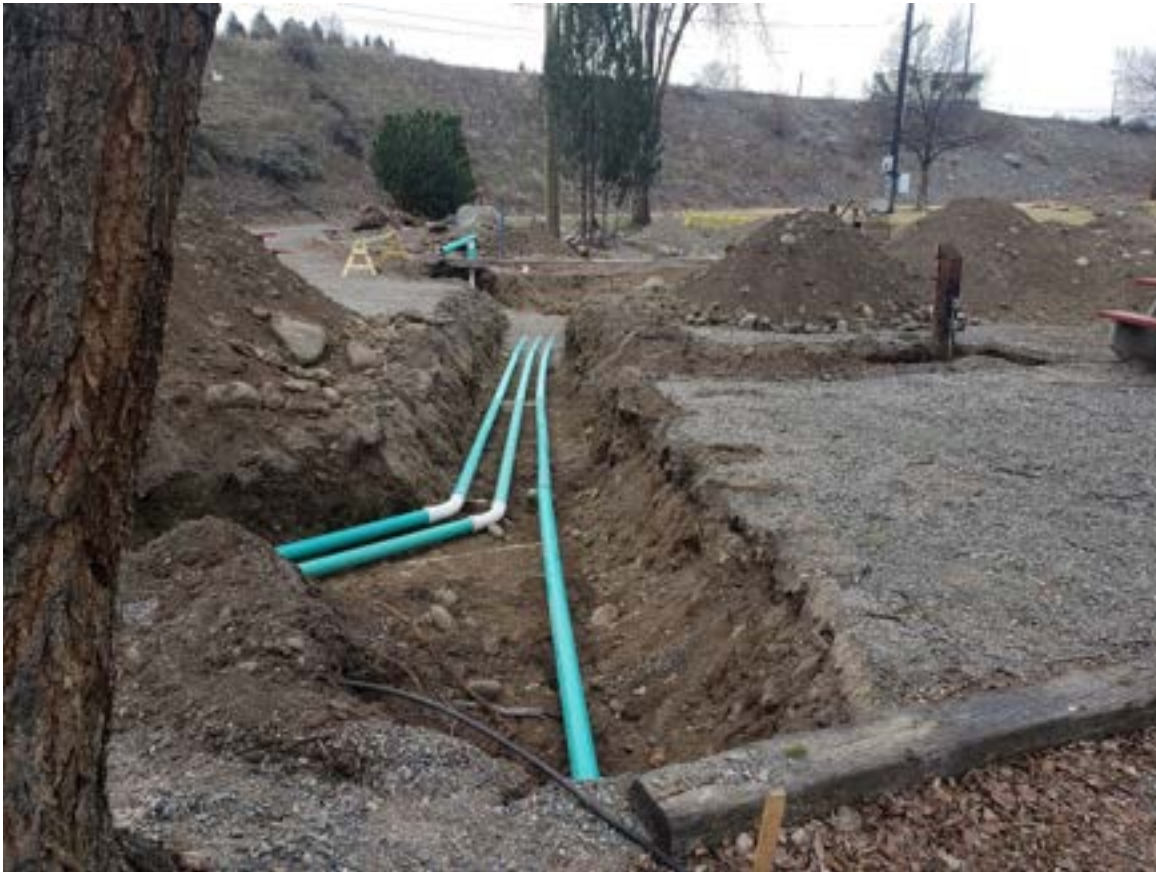
New sewer lines at Legacy Park
