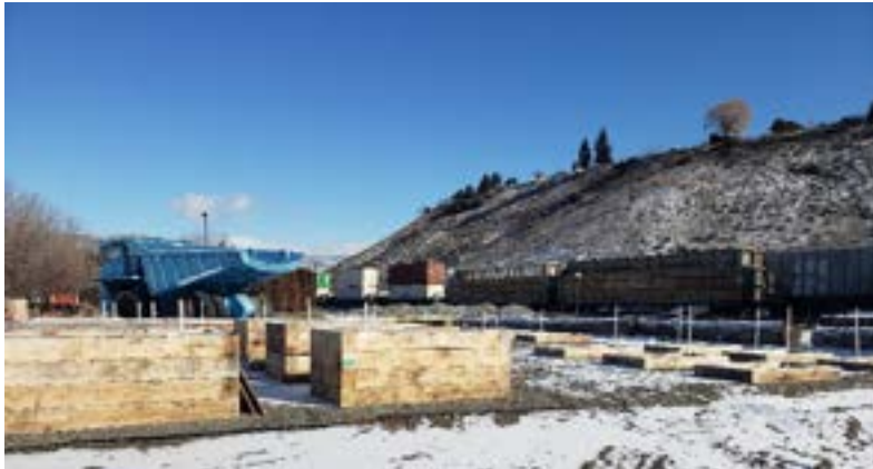
Left – Community Garden under construction.
