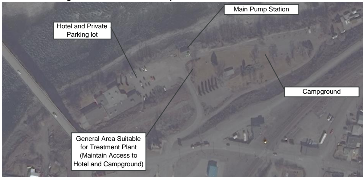
Figure 4.2: Overview of Pump Station and Treatment Plant Area
