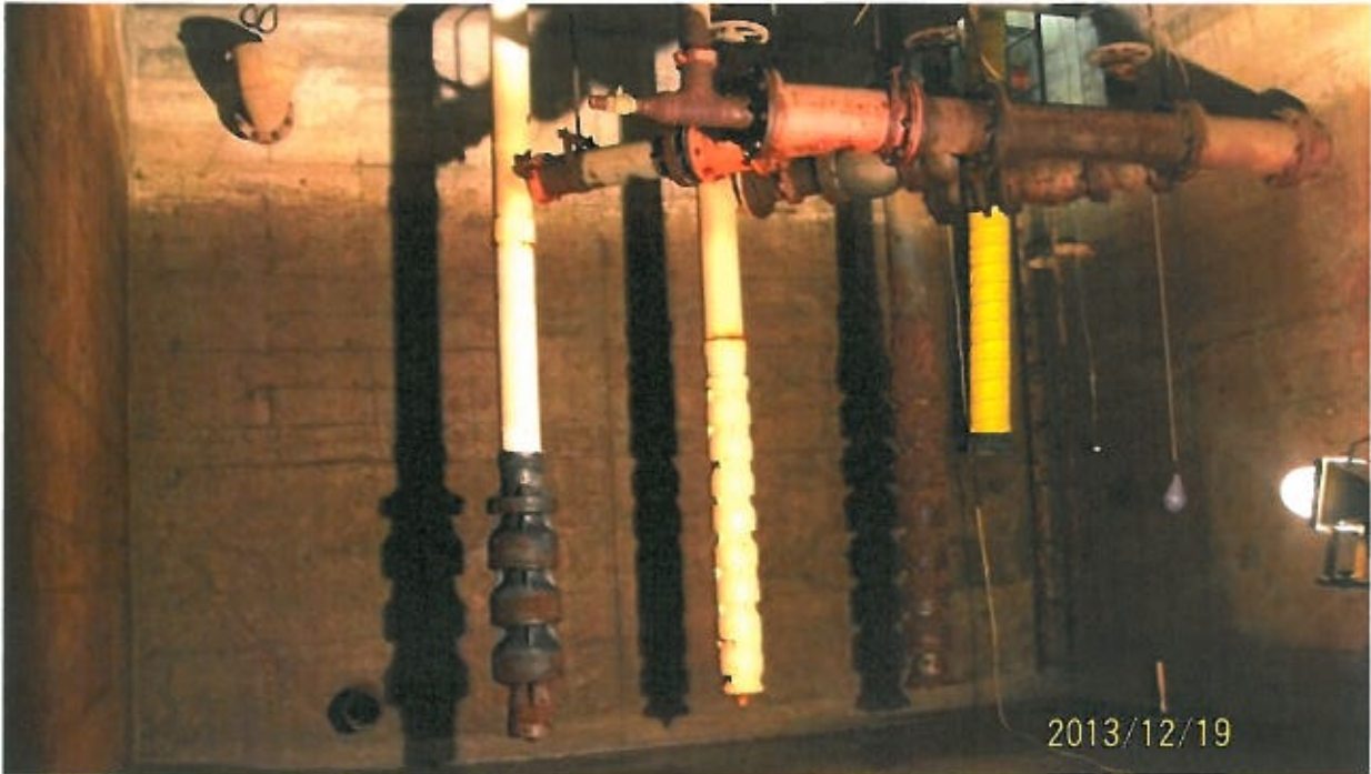
Photo 31 (Zone 3 Pump Chamber)
