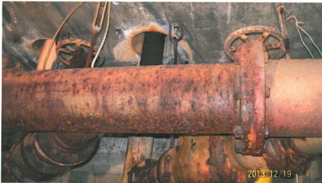
Photo 30 (Zone 3 Pump Chamber)
