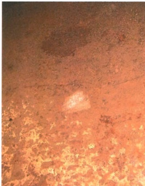
Photo 28 (Zone 3 Pump Chamber)
