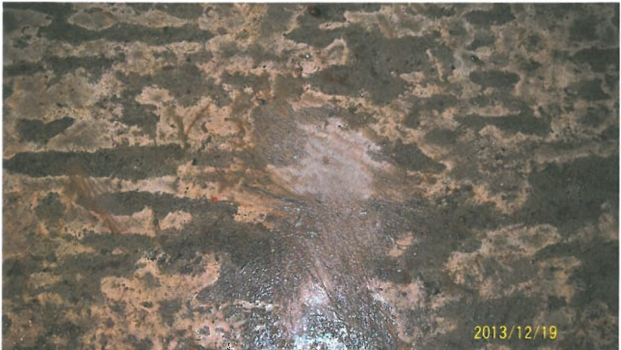
Photo 27 (Zone 3 Pump Chamber)
