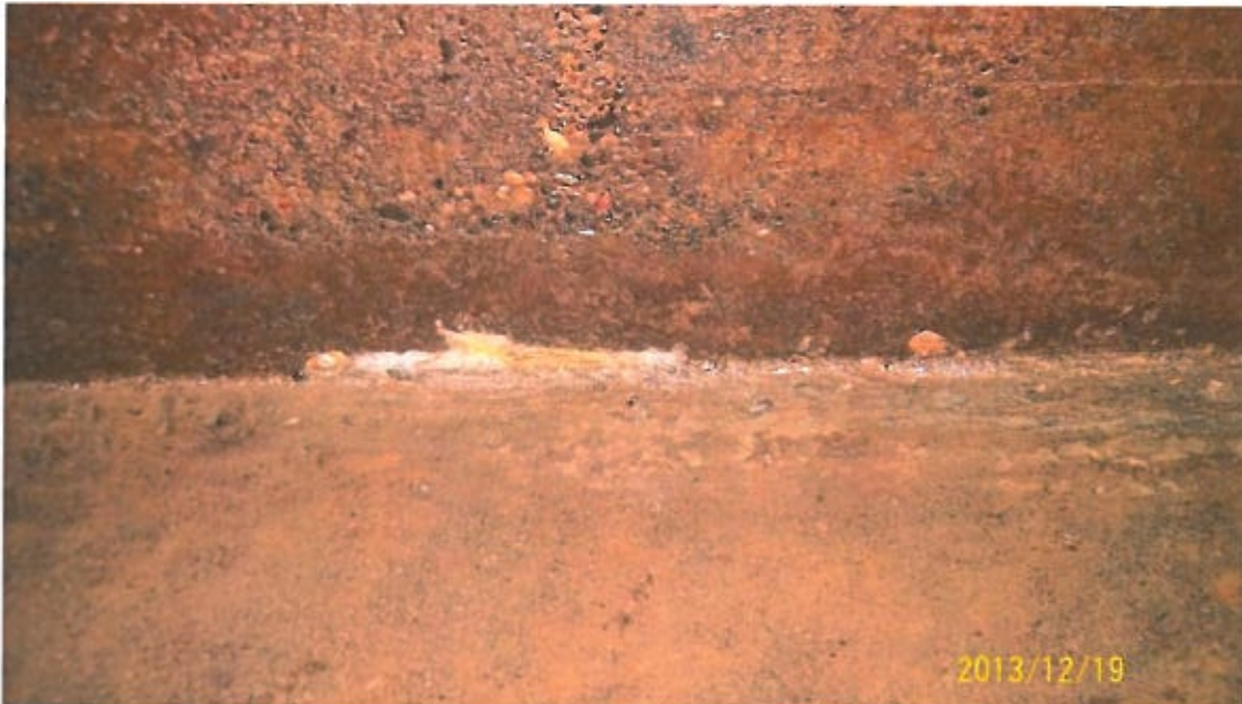
Photo 26 (Zone 3 Pump Chamber)
