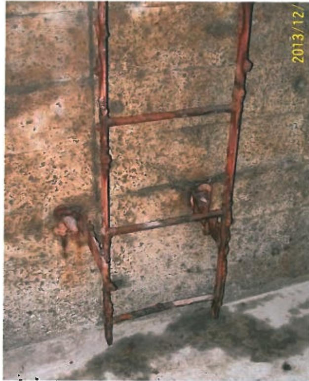
Photo 29 (Zone 3 Pump Chamber)
