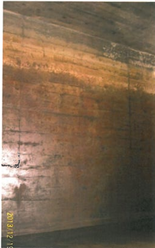
Photo 22 (Zone 3 Pump Chamber)
