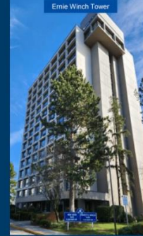
Ernie Winch Tower
